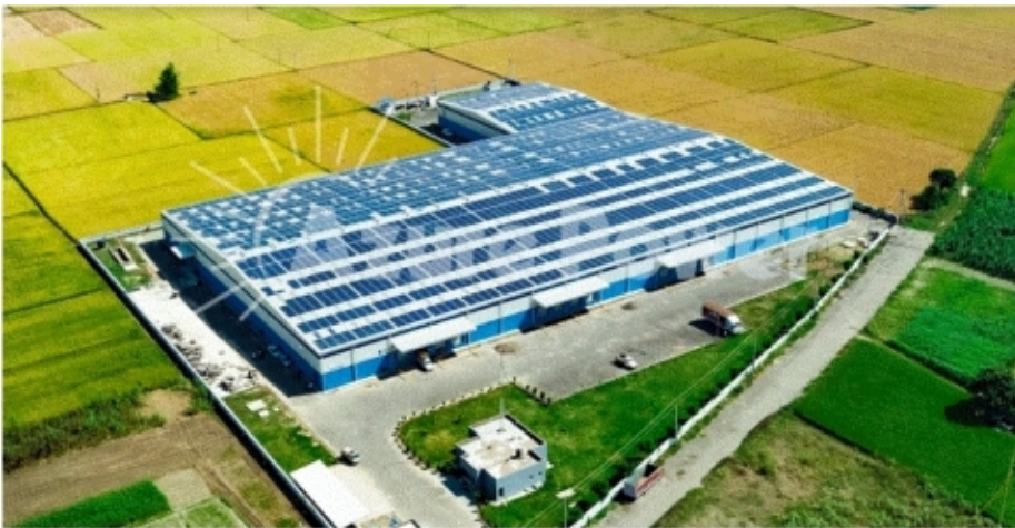
Azure Power Solar Rooftop Plant (Photo: Business Wire)
