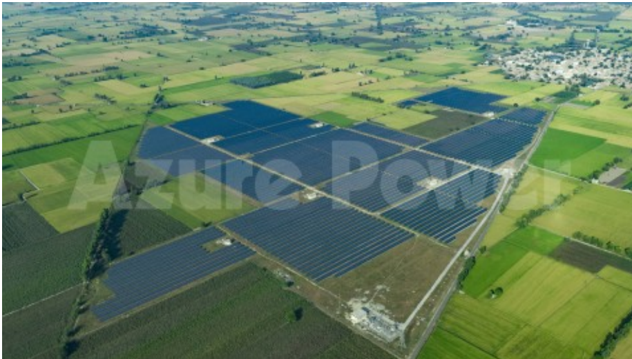
Azure Power Solar Plant (Photo: Business Wire)
