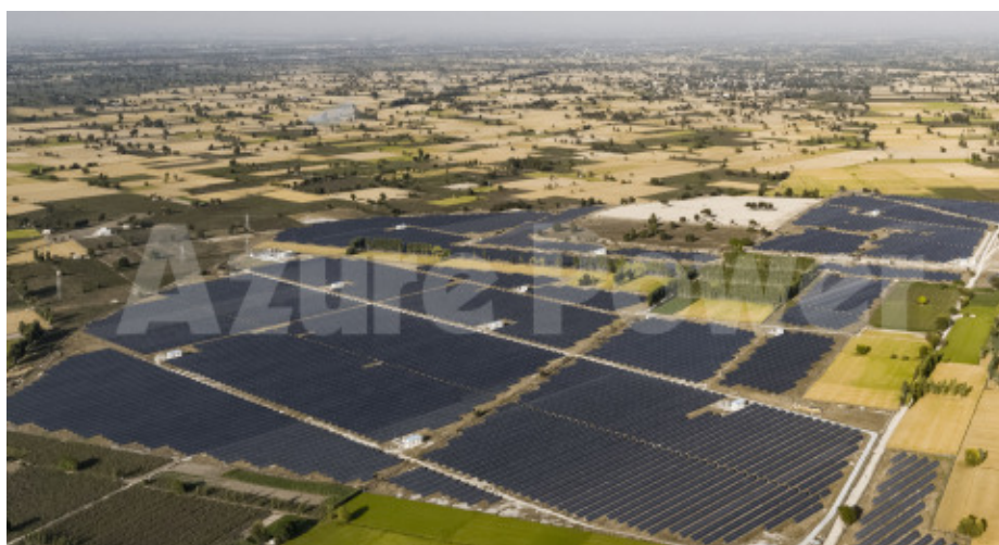
Azure Power Solar Plant (Photo: Business Wire)
