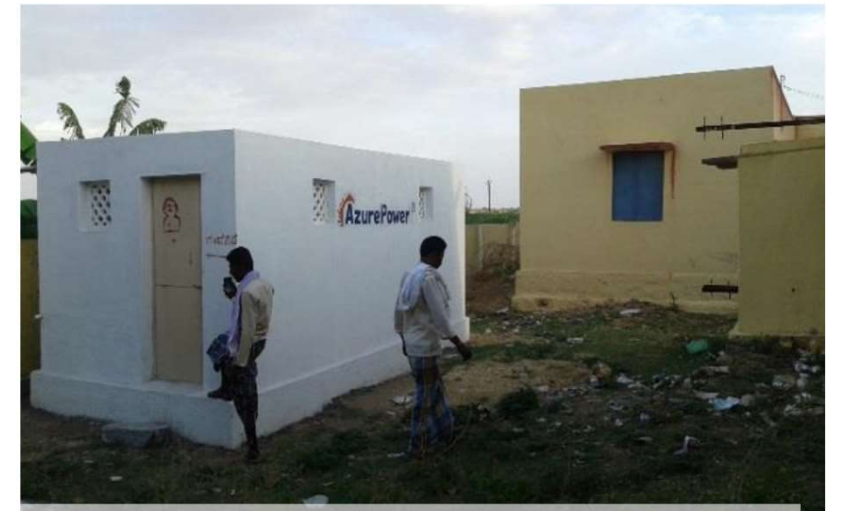
Built community toilets for sanitation and hygiene
