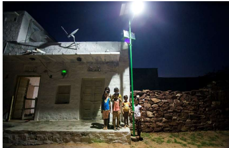
1,000+ Solar street lights installed to promote rural electrification
