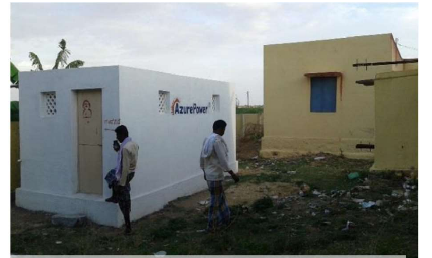
Built community toilets for sanitation and hygiene
