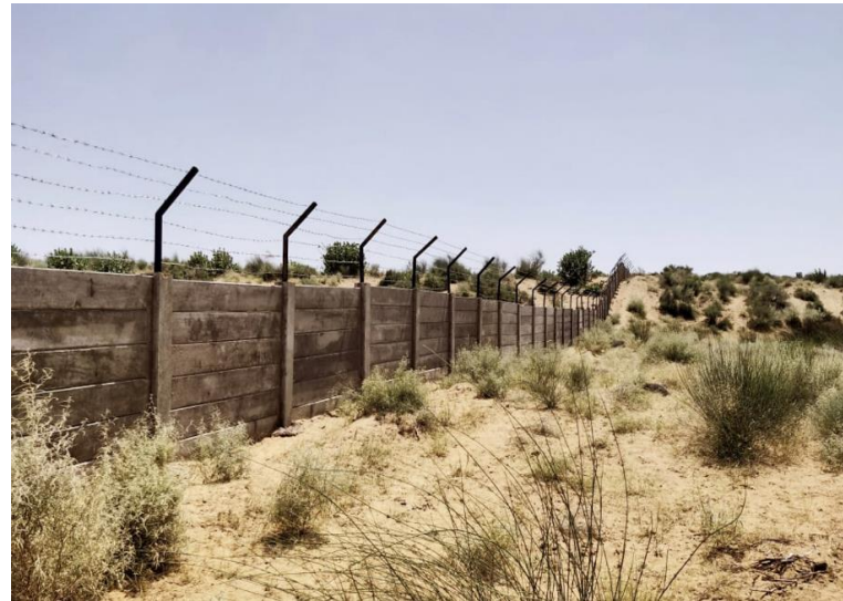
Fencing and piling under progress
