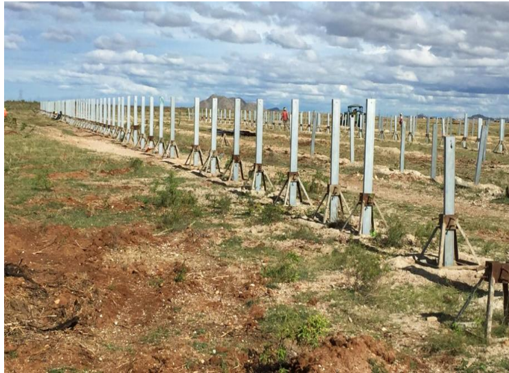
Fencing and piling under progress
