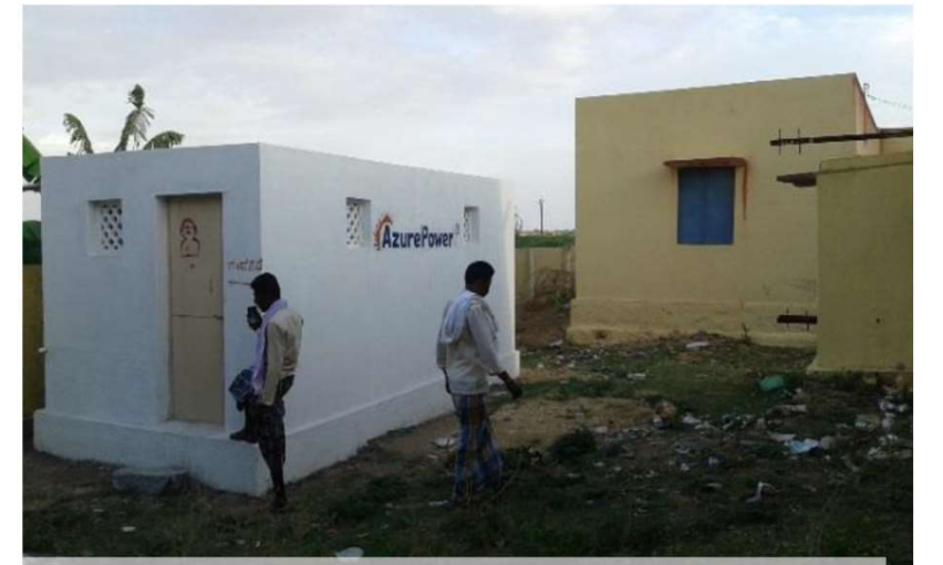
Built community toilets for sanitation and hygiene
