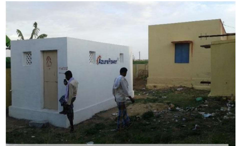
Built community toilets for sanitation and hygiene
