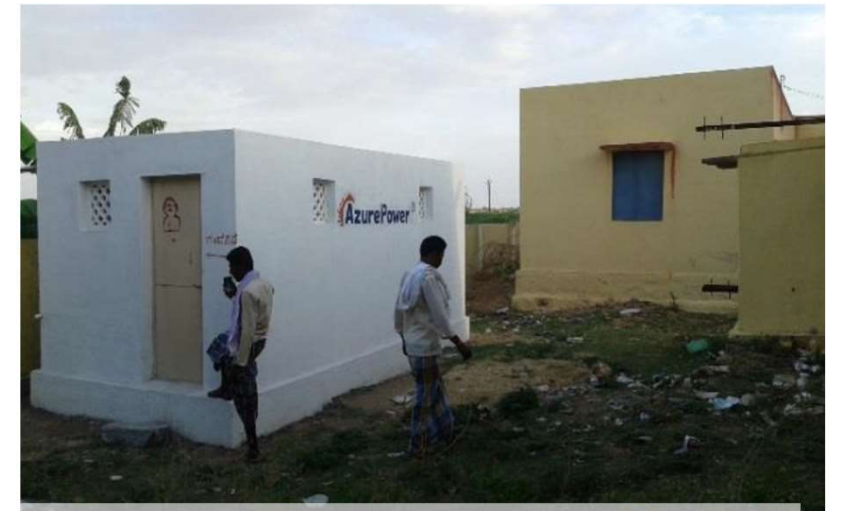
Built community toilets for sanitation and hygiene
