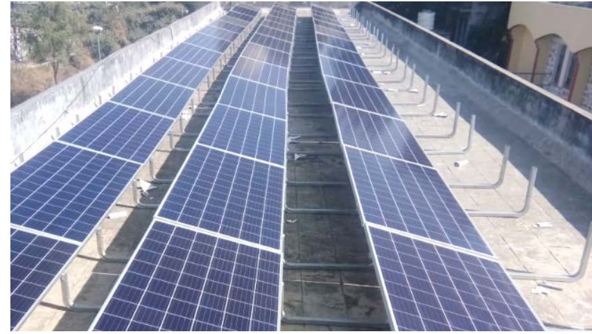
Rooftop project under construction
