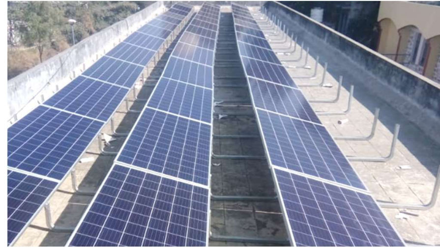
Rooftop project under construction
