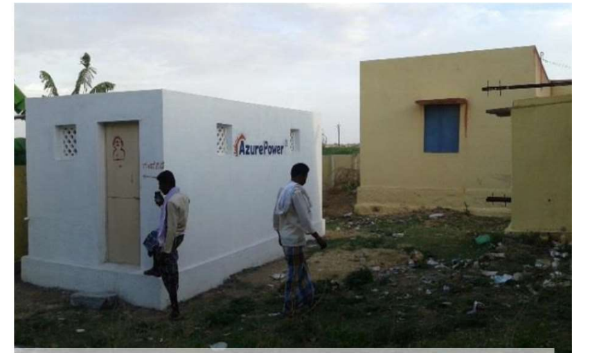
Built community toilets for sanitation and hygiene
