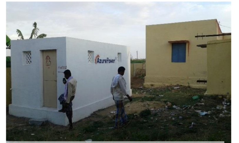
Built community toilets for sanitation and hygiene
